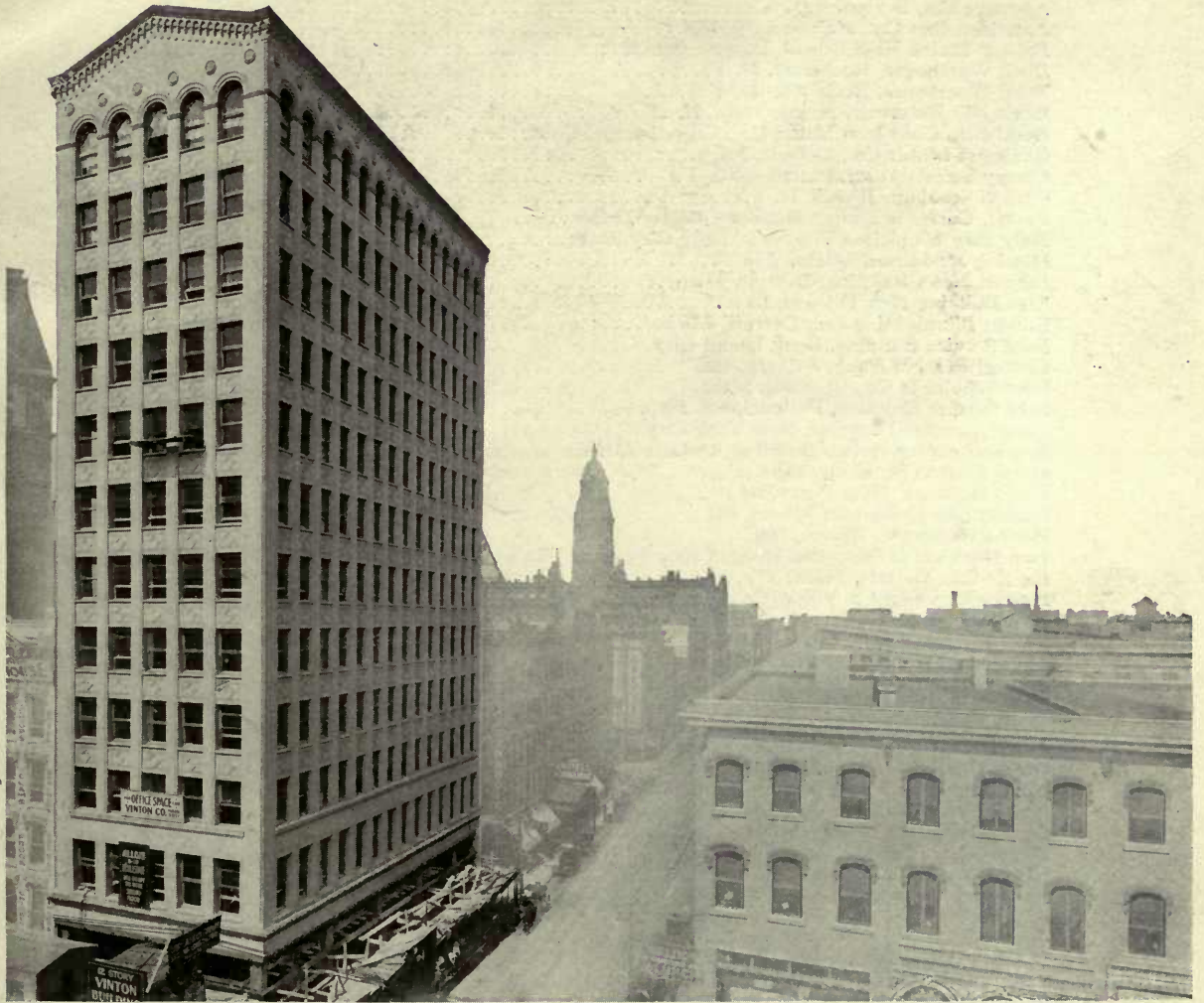
Vinton Building, Detroit, Michigan. Albert Kahn, Architect, Ernest Wilby, Associate Foundations waterproofed with Truscon Waterproofing Paste, Concentrated.
